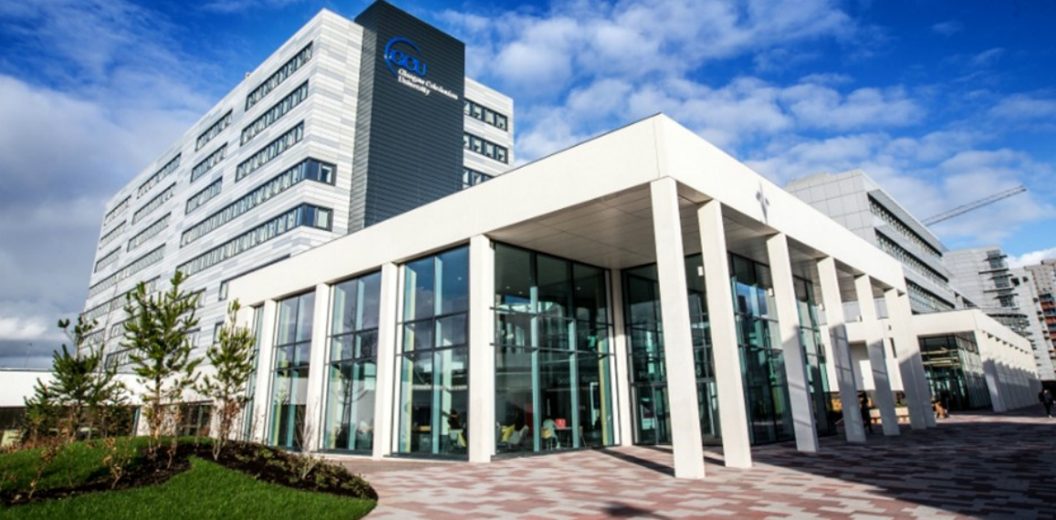
GCU Campus – Annie Lennox Building
